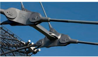
The advanced corrosion protection begins with corrosion protection category **C3 (moderate corrosivity).** In this case, 2-component products are mainly used, which meet the increasing requirements.
