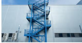
The corrosivity category **C5 (very high corrosivity)** stands for a very demanding corrosion protection at the highest level. 2-component paint systems are used almost exclusively to achieve high coating thicknesses.
