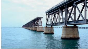
The corrosivity category **C4 (high corrosivity)** requires high performance from the paint components used. For these areas, basically 3-layer coating structures are applied. In case of 2-layer systems, only high-build coating structures are used.
